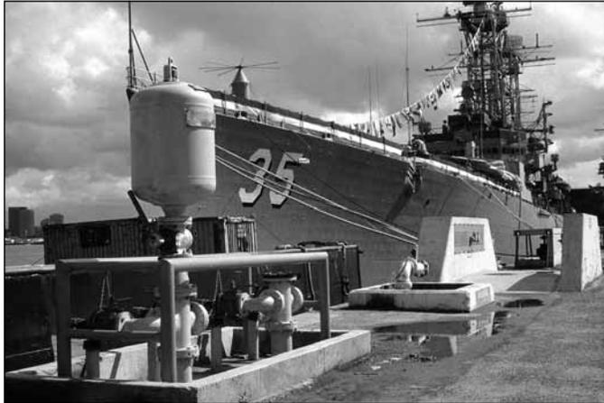
**Fuel loading absorbs shock from pump startup and stopping**
